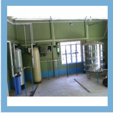
Safe Drinking Water Turnkey Project
